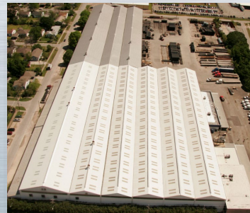
Merfish Pipe & Supply Houston, TX
